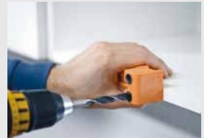
For drilling assembly, the TIP-ON unit is drilled in the centre of the cabinet base.
